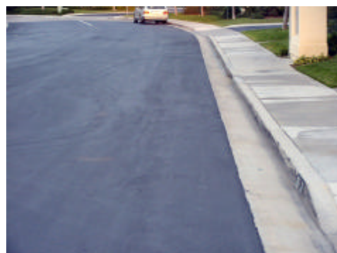
Same street with no water in the gutter.
