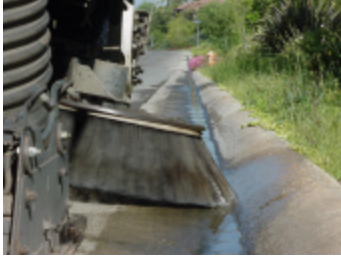
Gutter broom at work.
